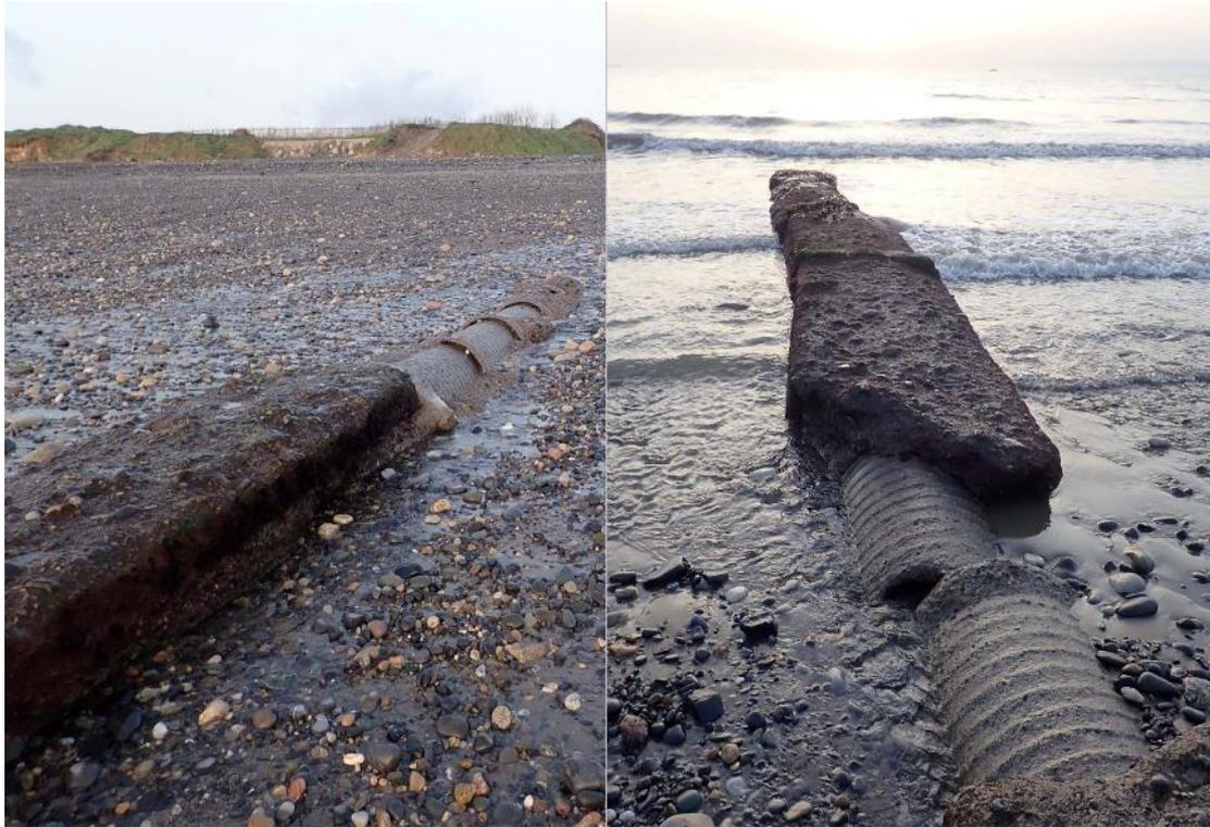
Figure 3.13: Storm flow discharge pipe in shore below Shanganagh WWT.
